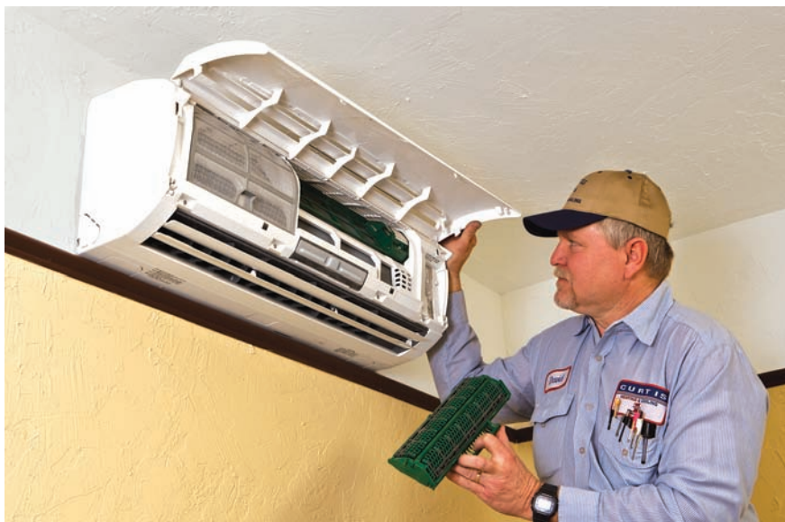
David Conner, service manager and tech adjusting air circulation and reinstalling a Fujitsu air filter.
