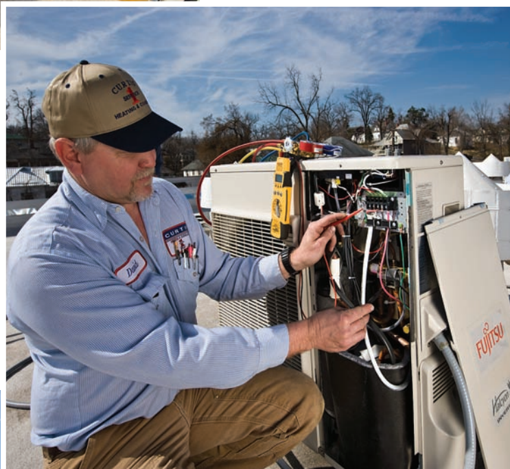
(TOP) David Conner, checking proper voltage as Cash Curtis checks a separate unit while Philip Curtis looks into another unit's refrigeration line set. (RT) David Conner, checking unit out.
