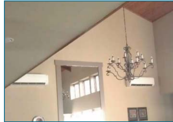
Two wall mounted ASU18RLF indoor models shown in the great room.
